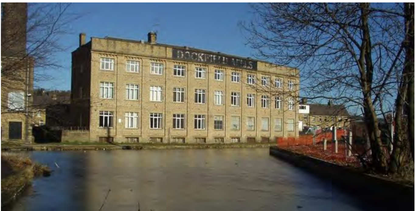
The remains of the Bradford Canal where it joined the Leeds and Liverpool Canal
